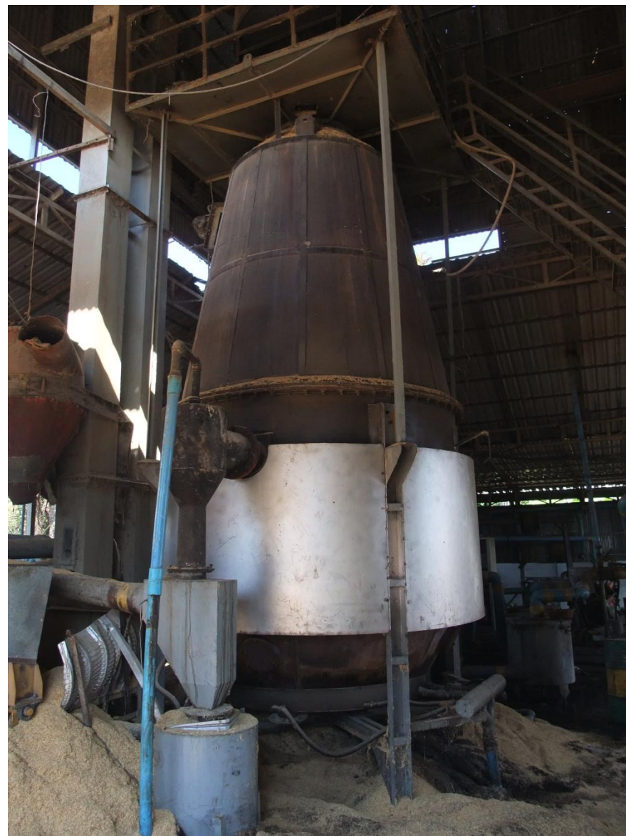
600kW gasifier, local manufacturer at Yam Chan rice mill, Battambang province, Cambodia, KH. 2014 - 12 - 20
