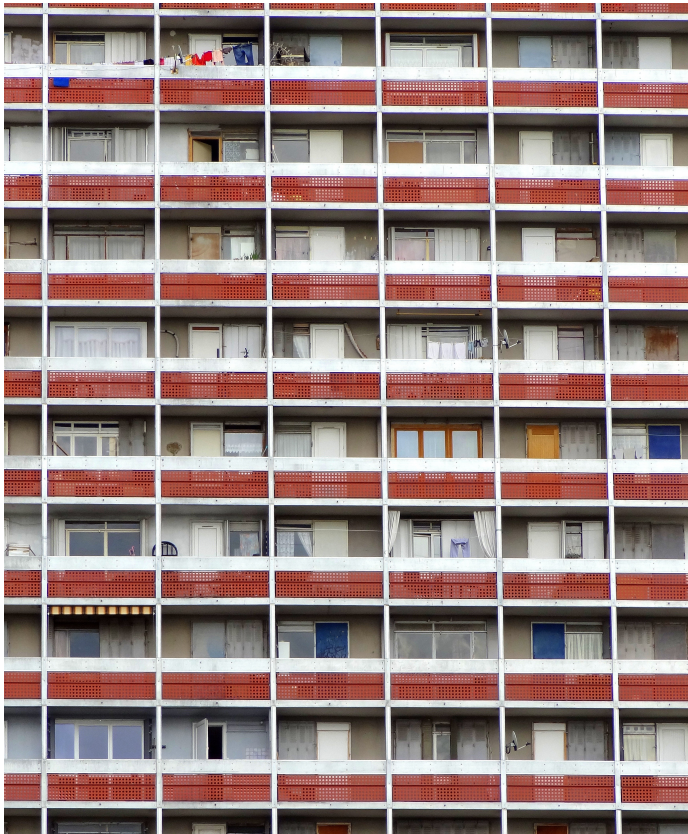
Figure 1- Housing Unit Marseille, photographer Bernard Lafond
