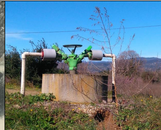
A pump under pressure
