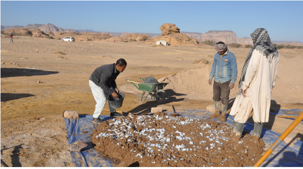
Fig. 3. Preparation of the mud mortar in 2017.
