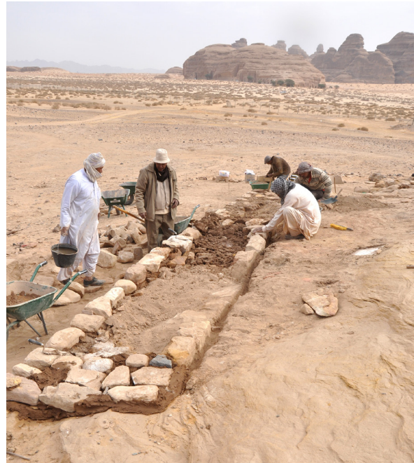
Fig. 4. Wall 60882 during restoration of the masonry.
