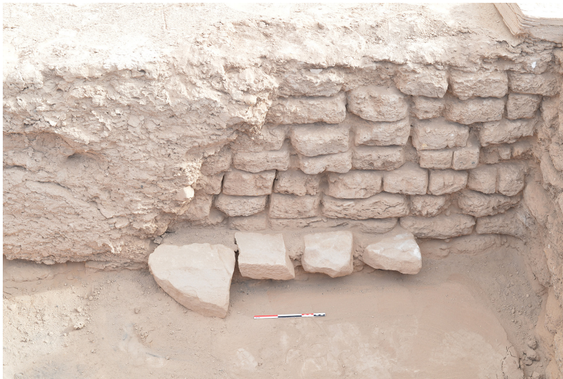
Fig. 11. Tower 12, interior, wall 35003 in the process of being scraped down to the mud-brick masonry. Leaning against the base of the wall are the remains of what was identified as paving (35363). Looking north-east.
