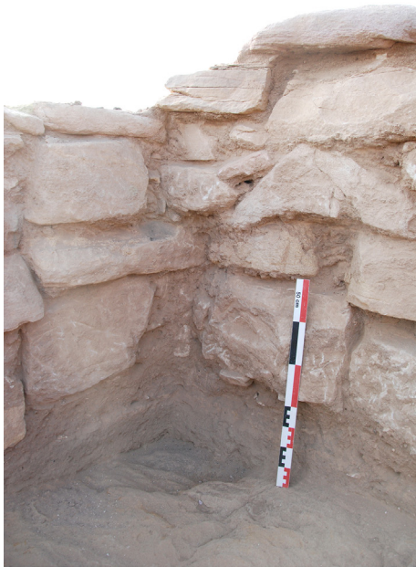
Fig. 16. Joined corner of the temenos wall (60809/60810) laid on top of the construction fill 61041.
