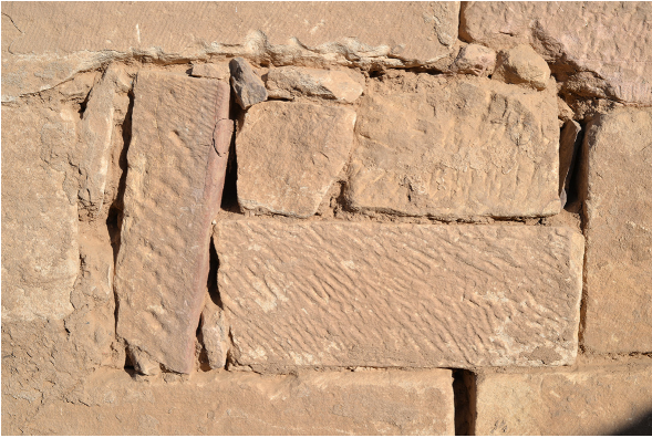
Fig. 24. Sounding H deep. Detail of the masonry of the foundations of wall 35002 (second state of the gate, facade wall of Tower 13): the evident fill (35332) of a cavity, marks left by extraction tools on the de facto lintel of the cavity. Looking north-west.
