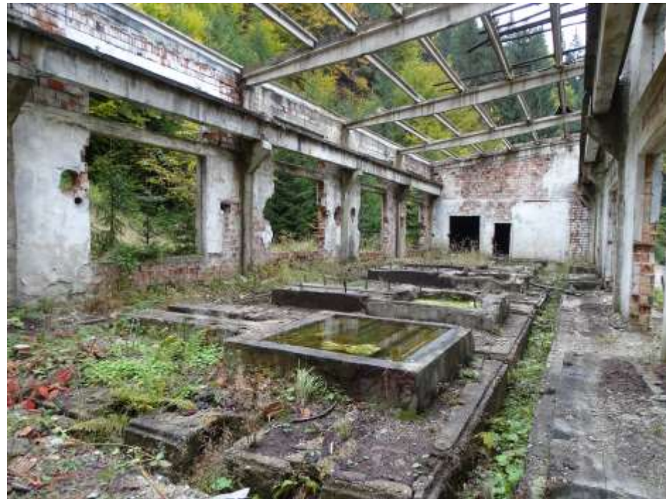
Ruined industrial building © V. Py
