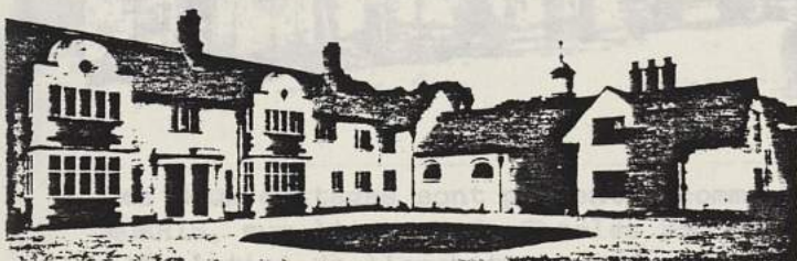
"GREYSTOKE," NEAR WARWICK: THE STABLES
