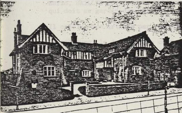
BOURNVILLE: COTTAGES IN LINDEN ROAD (FRONT VIEW)
