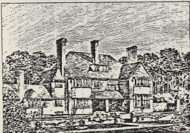
HOUSE AT SUTTON COLDFIELD
