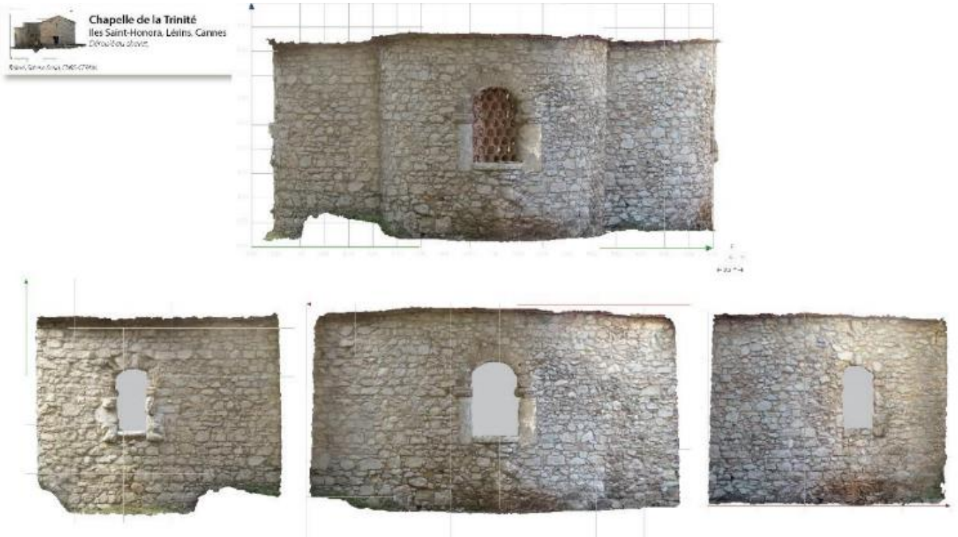
Figure 9: Orthoimage developed from the 'chevet' of the Chapelle de la Trinité – Iles Saint-Honorat, Cannes (France) – S. Sorin/CEPAM
