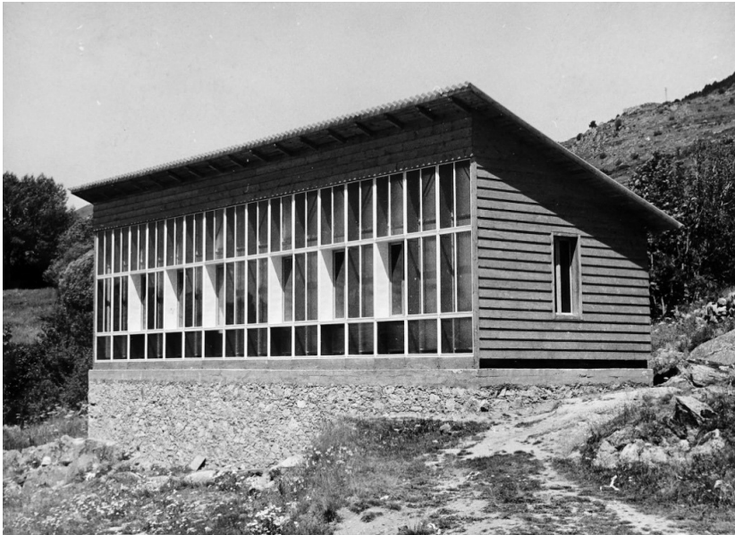
Figure 5: Experimental solar house, Odeillo, France, 1962-1963. South façade with Trombe wall.
