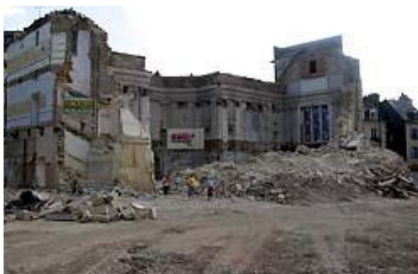
Picture 7: Rennes: Construction of a shopping center in the inner fringe belt.
