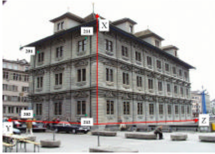
Figure 9. Local coordinate system and control points
