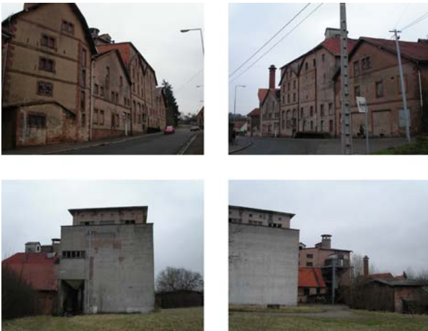
Figure 3. Ingwiller old malt house
