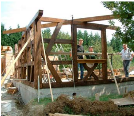
Figure 1. First stage in the construction of an Alsatian half-timbered house
