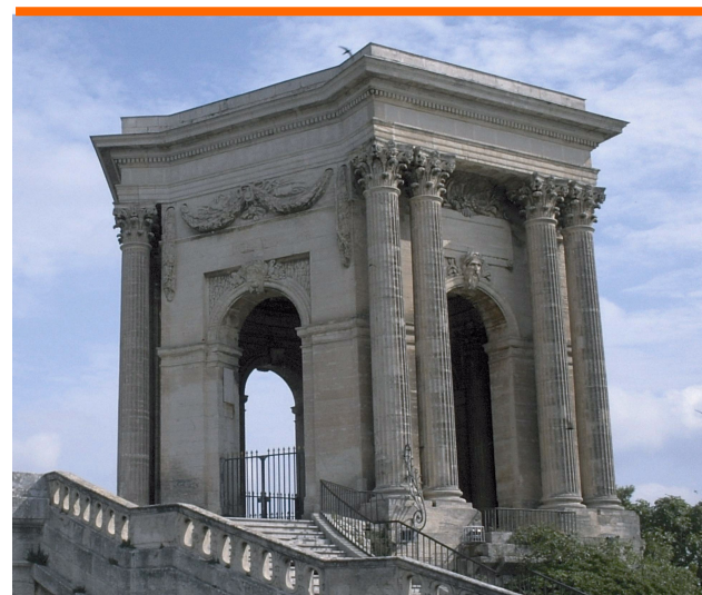
Figure 5. The Water Tower
