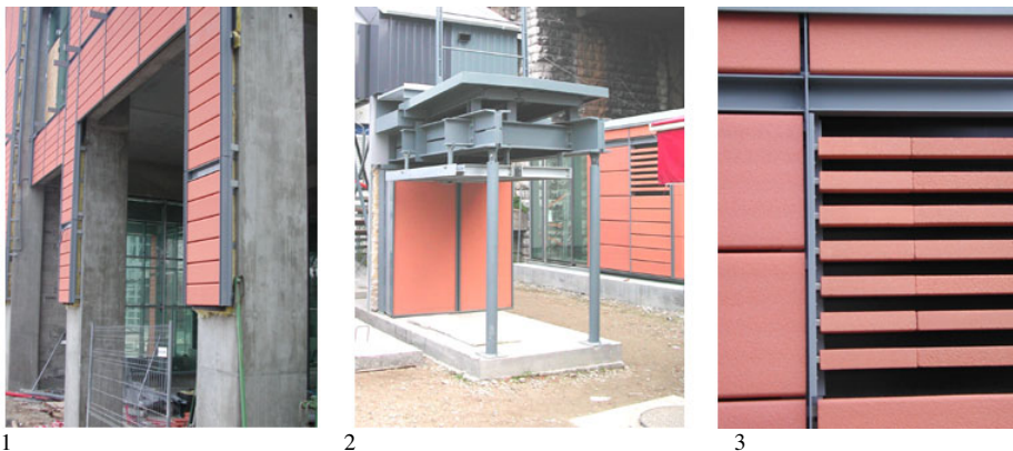
1 Building site of the Cité internationale in Lyon and experimental prototypes. Photo N° 3 : variations of the brick component.
