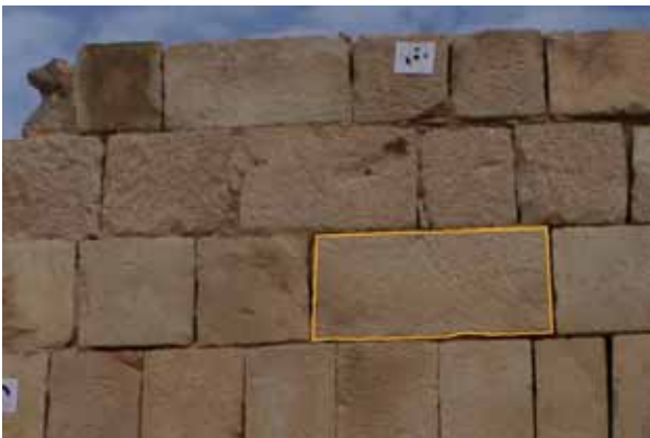
Figure4: A block perimeter easured with Arpenteur
