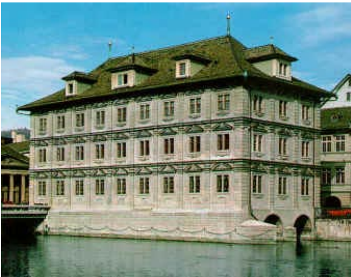
Figure 1: Zurich city hall (seen from southwest).
