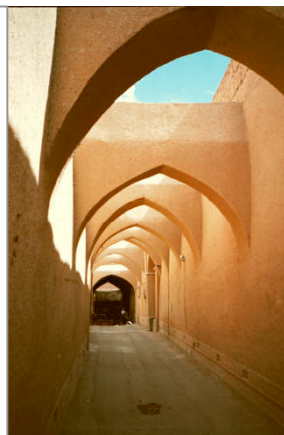
F.3: The narrowness of the semi-covered passageways and high walls along two sides of allays make shade in summer afternoons and protect the complex against the dusty desert winds.
