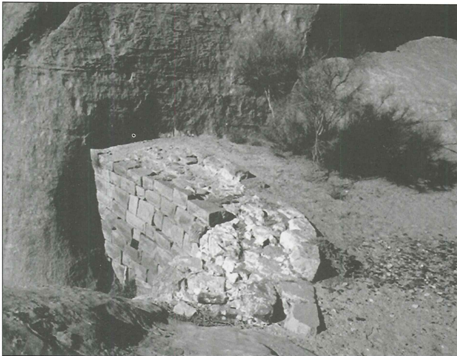
6. Umm Daraj retaining dam.
