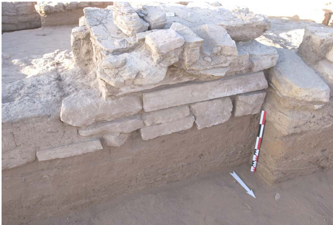
Fig. 4. The installation 20005 on top of stone substructure 20036 and the cut section of wall 20008 to the right
