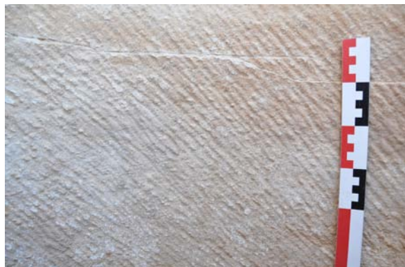
Fig. 61. Bottom of basin no. 1
