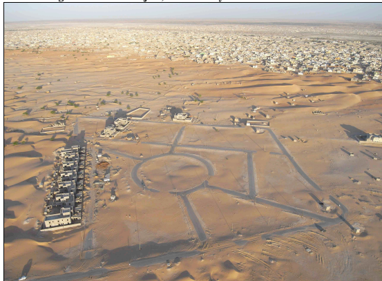
Fig. 4: “Sukuk” Project, in the sandy outskirts of Nouakchott
