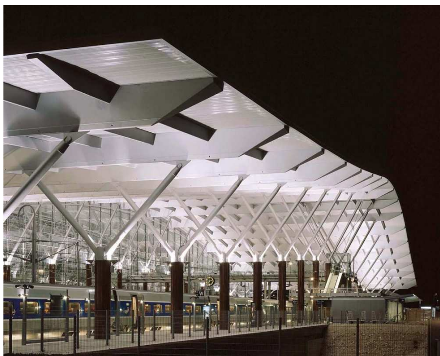
FIGURE 10: GARE D'AIX-EN-PROVENCE TGV. SOURCE: AREP.
