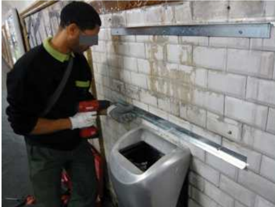
Figure 7. Drilling. © Photo: J. Denis and D. Pontille.
