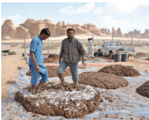
Fig. 13.10 Trampling the earth with the temper
