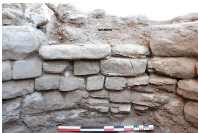
Fig. 49 The overflow rests on a stone which is slightly protruding from the masonry
