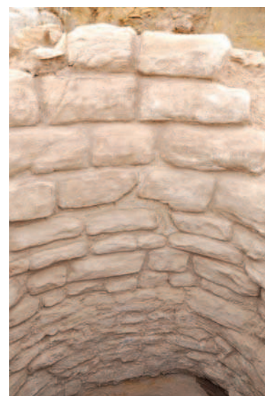
Fig. 46 The masonry of the well on the western side. Note the size of the ashlar, which are much larger at the top than at the bottom
