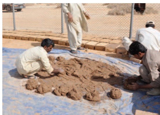
Fig. 13.13 Clods of earth prepared for the filling of the mould
