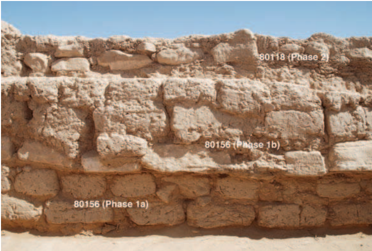
Fig. 12 Phase 1a and 1b of wall 80156, and wall 80118 belonging to Phase 2
