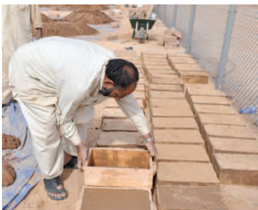
Fig. 13.16 Removal from the mould
