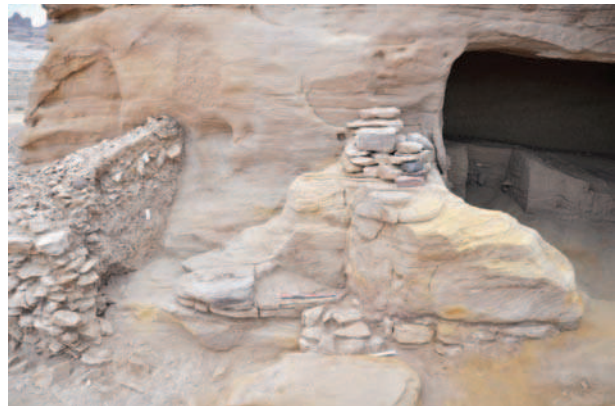
Fig. 8 Part of the ramp which was installed to the left of the rock-cut chamber IGN 132a after the ceiling collapsed
