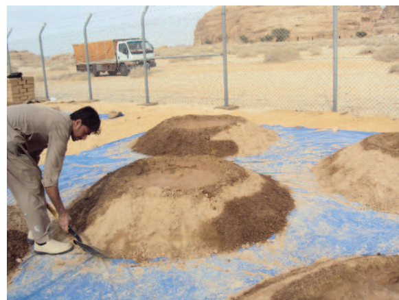
Fig. 13.6 Bringing the earth up on following morning
