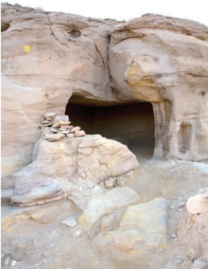
Fig. 7 View of the rock-cut chamber IGN 132a showing the collapse of the ceiling
