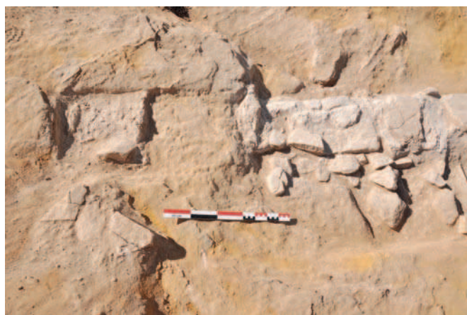
Fig. 11 The building techniques used for the western enclosure wall on top of IGN 132: the blocks and wedging stones make the best possible use of the bedrock and carefully follow its level
