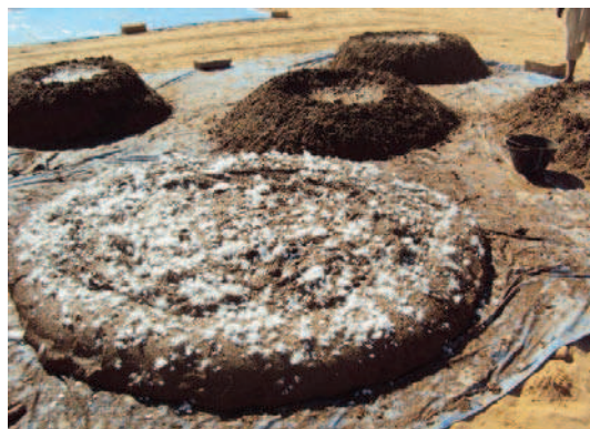
Fig. 13.9 Temper spread on top of trampled mound
