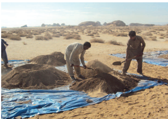
Fig. 13.4 Mixing of clay and sand with a shovel
