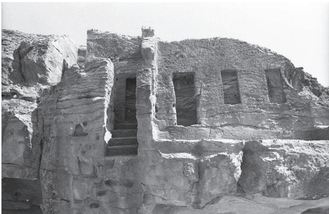
Fig. 72 The southern staircase leading up to the top of Dalman no. 520, from the west
