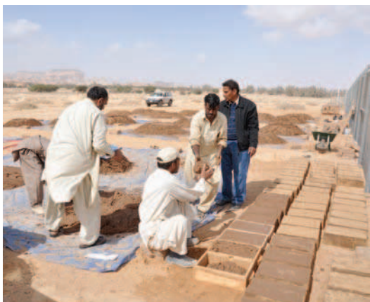
Fig. 13.14 Filling of the mould
