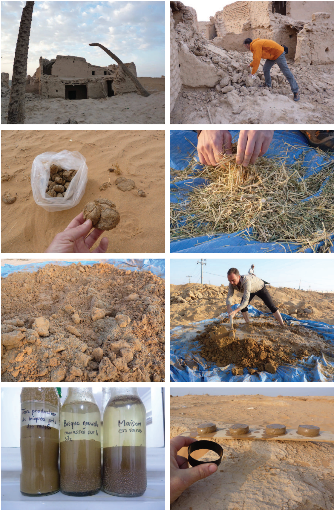
Photos illustrating the mortar preparation
