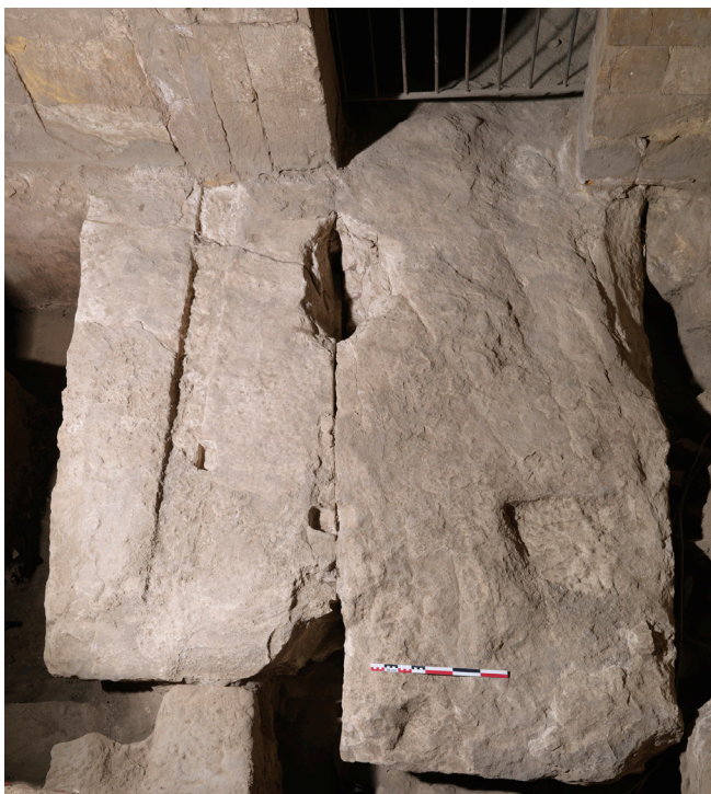
The central chamber with two limestone roofing slabs reused as pavement and foundation of the southern wall; the door at the top of the photograph leads to the south chamber. © CNRS-CFEETK/Jean-François Gout
