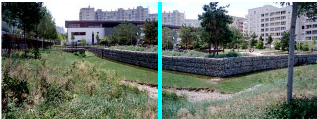
Figure 2. Photos of Jacob Kaplan Park. The detention basin is in the foreground (2011).
