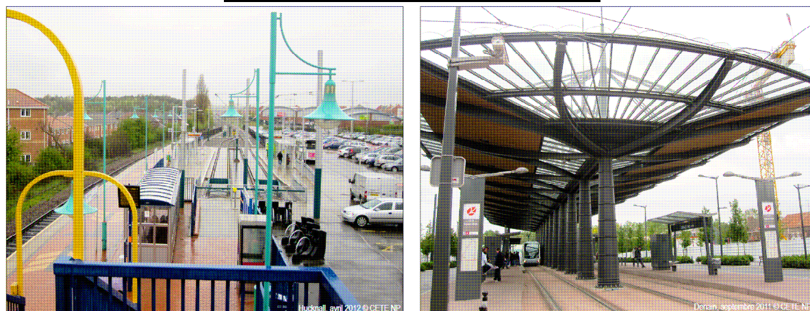
FIGURE 5. Terminal station in Hucknall and Denain
