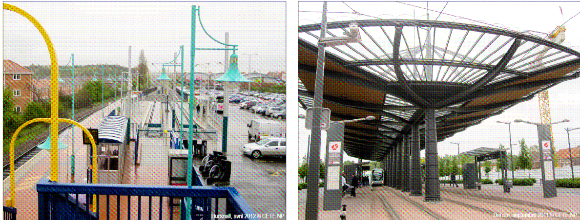
FIGURE 5. Terminal station in Hucknall and Denain
