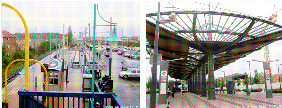
FIGURE 5. Terminal station in Hucknall and Denain
