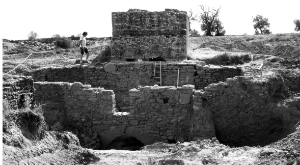
Fig. 4: The water mill of Palaiomylos
