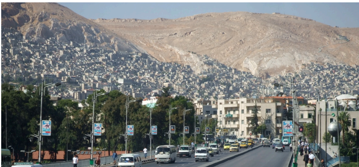
Figure 1- Informal settlements built on the slopes of mount Qassiu are overlooking the city centre of Damascus. Photo V.Clerc 2009.
