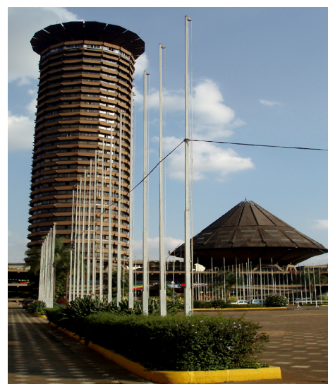
Photo 4.2 : The Kenyatta International Conference Centre (KICC), the tallest building in Nairobi at the time (author).
