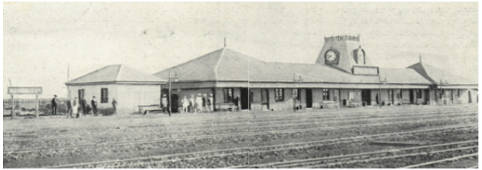
Photo 1.1: Nairobi Railway Station in 1906. Made out of mabati (corrugated iron sheets) and wood, this building has since been demolished (source: Railway museum).
