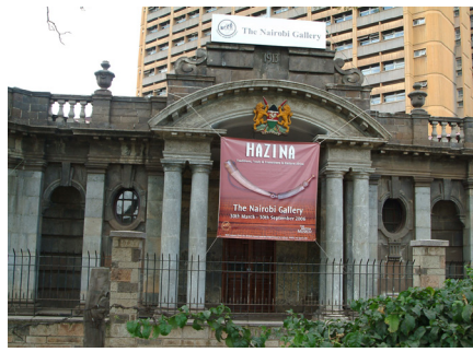
Photo 2.2: Built in 1913 for the Ministry of Native Affairs this building was later used as the D.C.'s, then P.C.'s office It now belongs to National Museums of Kenya
