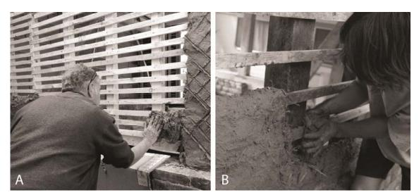
**Fig. 22.2** Various techniques of daub installation: (**a**) daub pressed against a closely spaced frame (with horizontal movements); (**b**) Elongated lump of daub set down on laths ("*torchis à cheval*"). Daub overlaps the horizontal element of the frame (picture: Parc naturel régional des Caps et Marais d'Opale).
