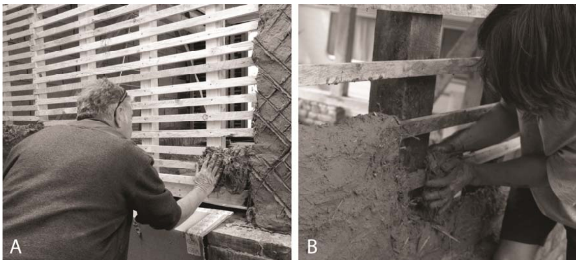
Fig. 22.2 Various techniques of daub installation: ( a ) daub pressed against a closely spaced frame (with horizontal movements); ( b ) Elongated lump of daub set down on laths (“ torchis à cheval ”). Daub overlaps the horizontal element of the frame (picture: Parc naturel régional des Caps et Marais d’Opale).
