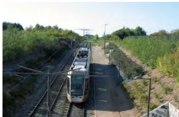
Illustration 29: tram platform ballasted - Orléans - source : AUAO
