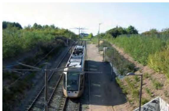
Illustration 29: tram platform ballasted - Orléans - source : AUAO
