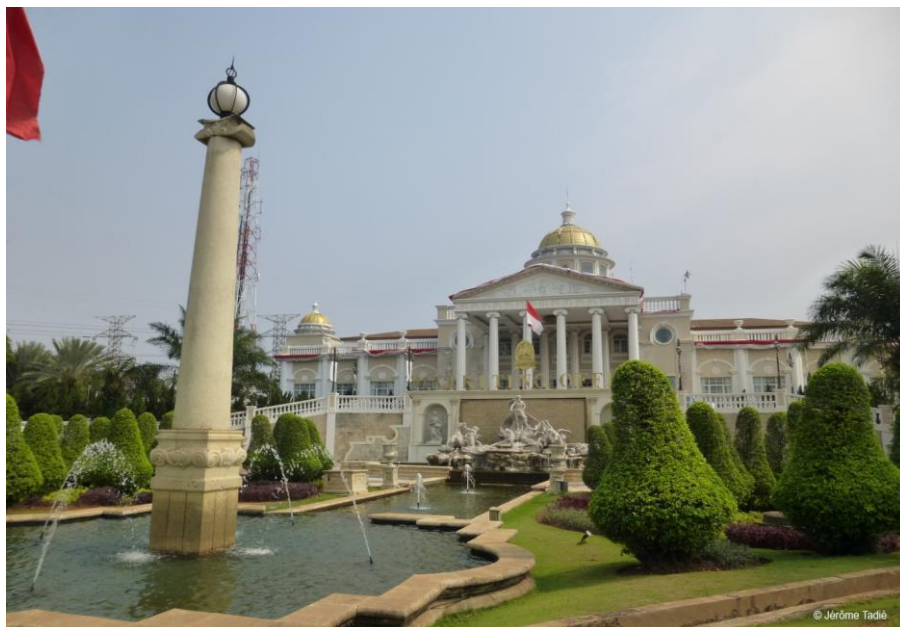
Figure 9: Boulevard Pantai Indah Kapuk
