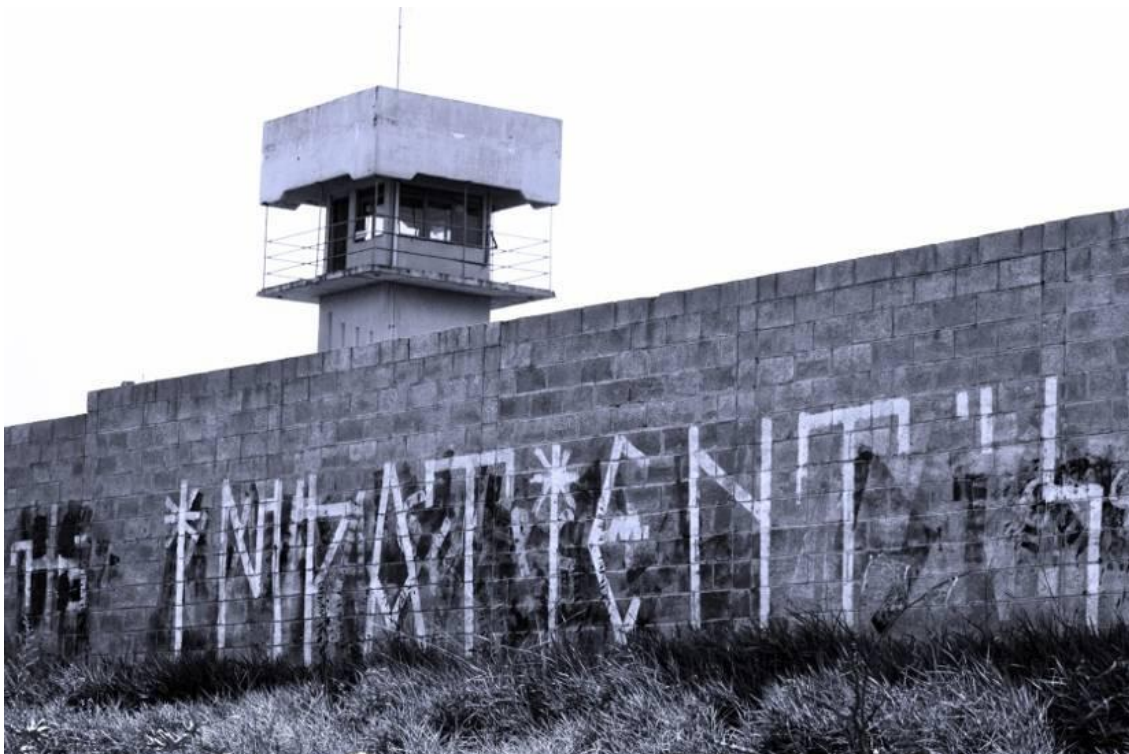
Figure 5. Façade of Campinas Prison, 2007. Photo: Tiago Macambira.
