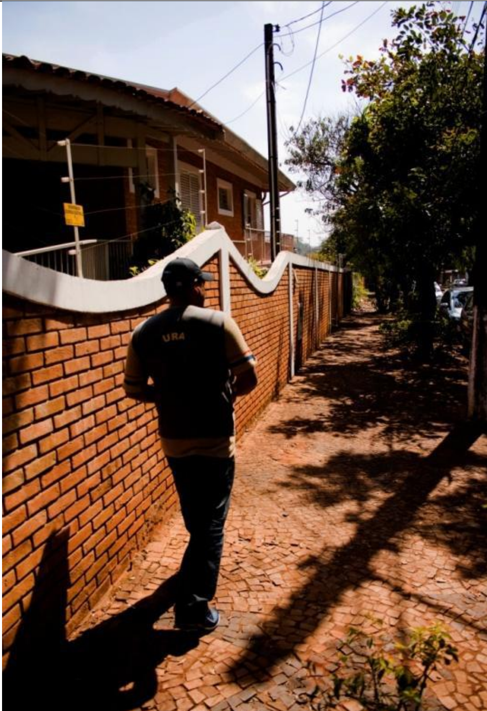
Figure 1. Non-compliant electric fencing in the Barão Gerlado neighborhood of Campinas, 2010. Author's photo.
