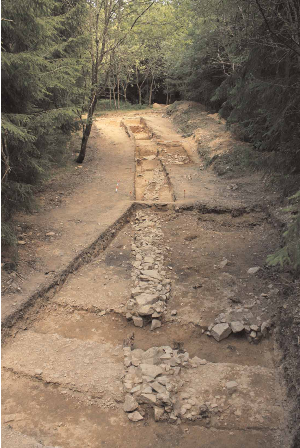
Figure 9. Photograph of drainage system from sondage 5. Photo: T. Moore.
