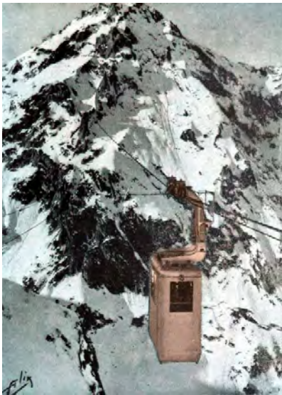
Three important steps in the history of the Pic du Midi observatory. The construction of the cable car, the construction of inter-ministerial building and the construction of the Bernard Lyot telescope.
