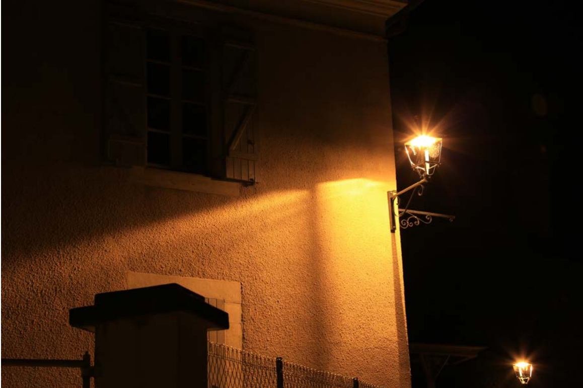
Main street of Geu. Full cut off lights; high pressure sodium lamps; 2200 °K; 8 lux.
