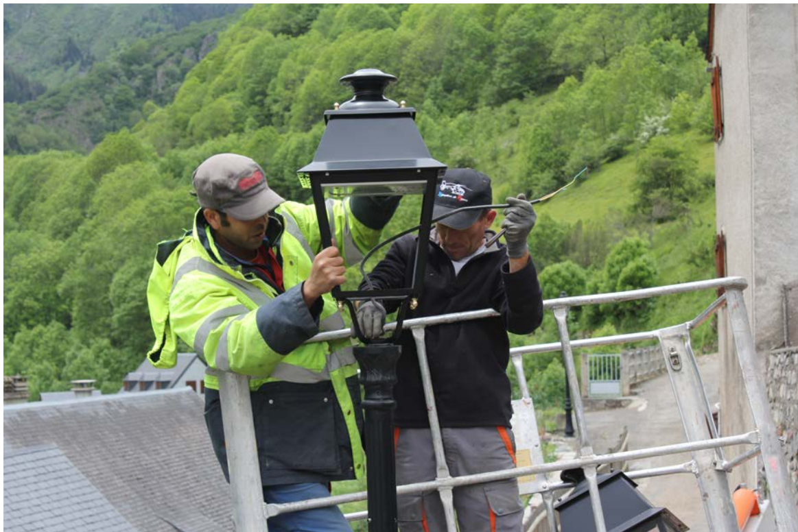
New generation of lantern, standard with the Lighting Guide of the Pic du Midi RICE/IDSR (Credits: Lea Salmon).
