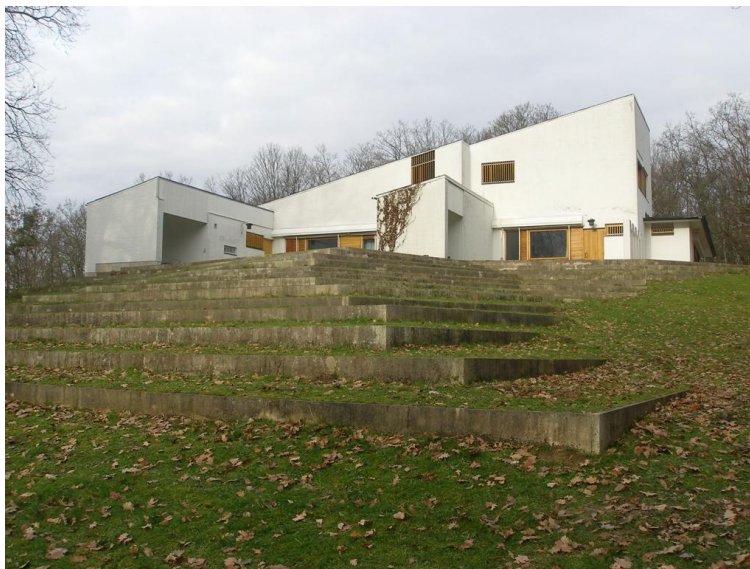
Maison Carré, Bazoches-sur-Guyonne (1956), the "turf stairs" create a transition between the house and the landscape.
