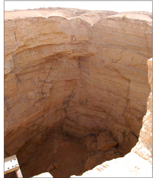
Figure 51 Sinkhole at ‘Ayn al-Ḍila’ 2 in 2011, looking southeast (photograph: J. Schiettecatte – French-Saudi Archaeological Mission in al-Kharj)
