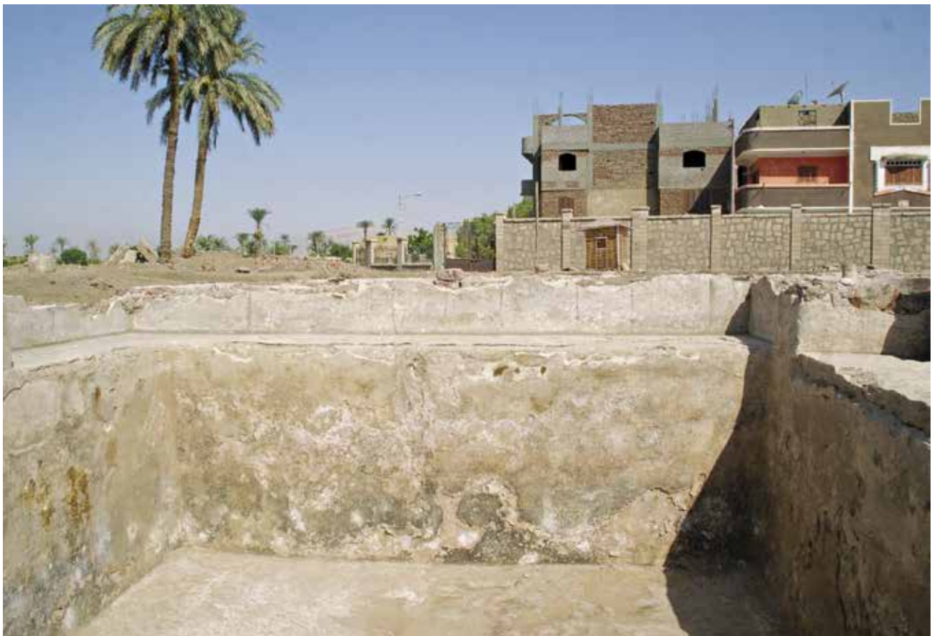
Fig. 11. View, westward, of the painted inside wall of Pool 10 (© P. Piraud-Fournet 2012).
