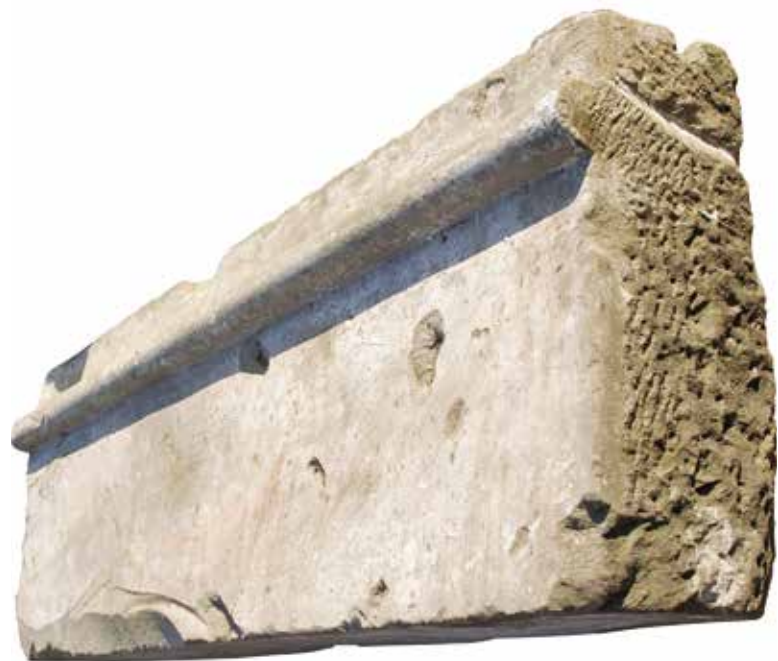
Fig. 5. Outer lintel of the front doorway of the baths (© P. Piraud, Fournet 2012).
