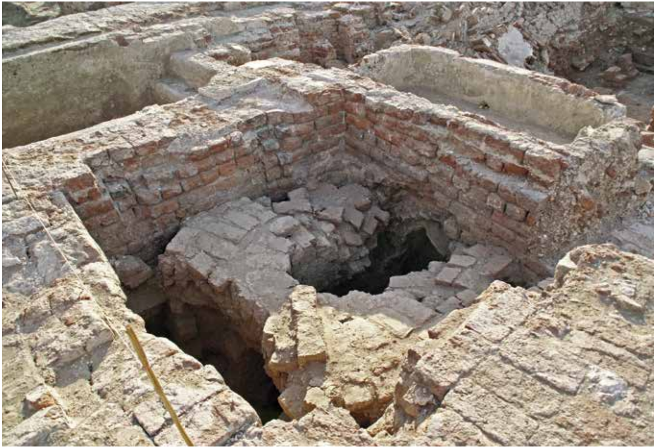
Fig. 20. View, north-eastward, of the structures containing Boiler 33 (© Th. Fournet 2012).
