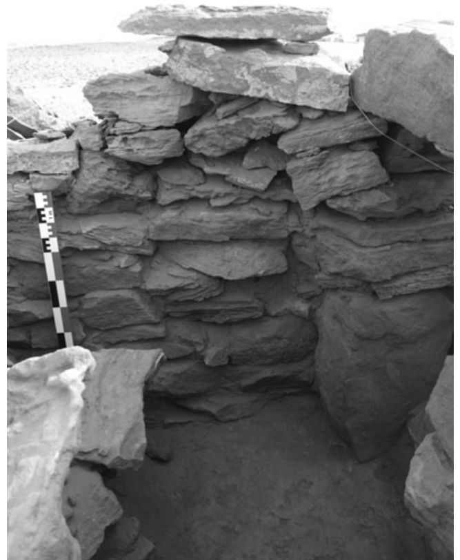
Fig. 14. Sector C, height of the wall.
