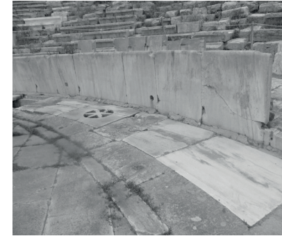
Fig. 10a, Opus signinum around the orchestra at the Theatre of Dionysus (Photo by author).
