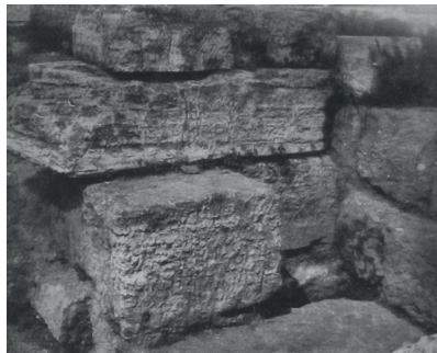
Fig. 7a, Foundations identified in the 1935 excavation as Roman, portion of wall RV the parascaenium (E. Fiechter, Das Dionysos-Theater in Athen , cit., fig. 26).
