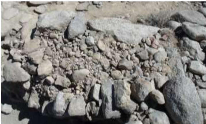
Fig.13: south-western wall (308, 309 and 310) from above ©MAFIL
