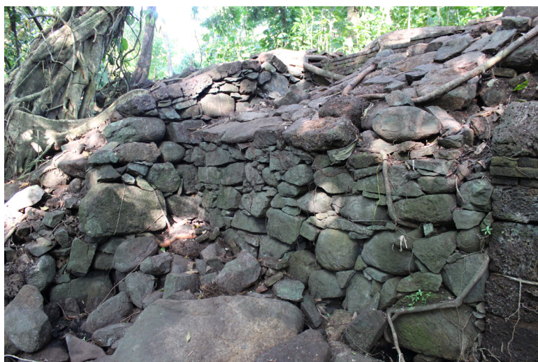
Figure 4 Glacis de moellons
