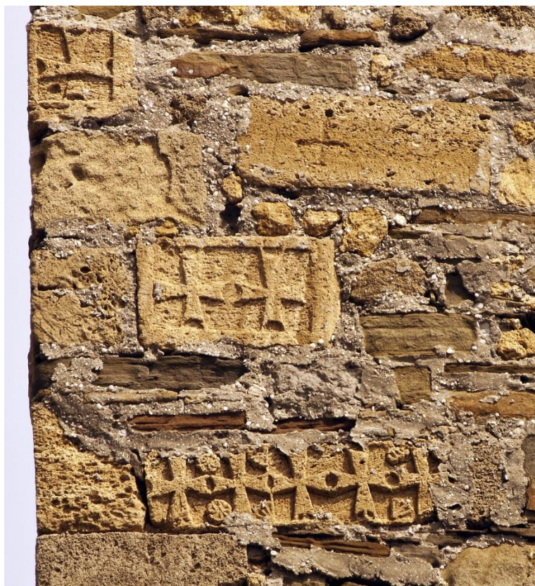
Fig. 18. Sudak. Tower of Federico Astaguera. South façade. Photo A. Dzhanov.
