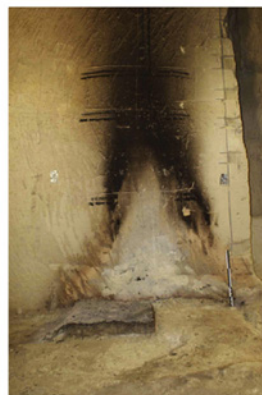
Fig. 12. Top: temperature distribution on a slice 20 cm in front of the wall of the fire (FDS) – bottom: rubification cone after the experimental fire in the quarry (credit: C. Ferrier).
